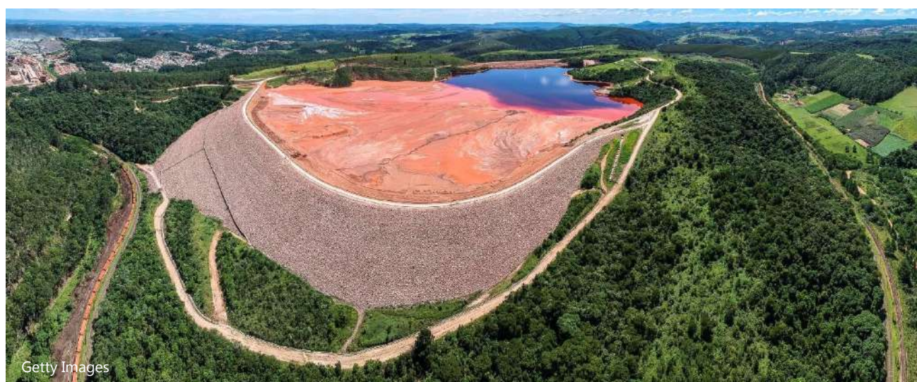
Tailings dam monitoring
